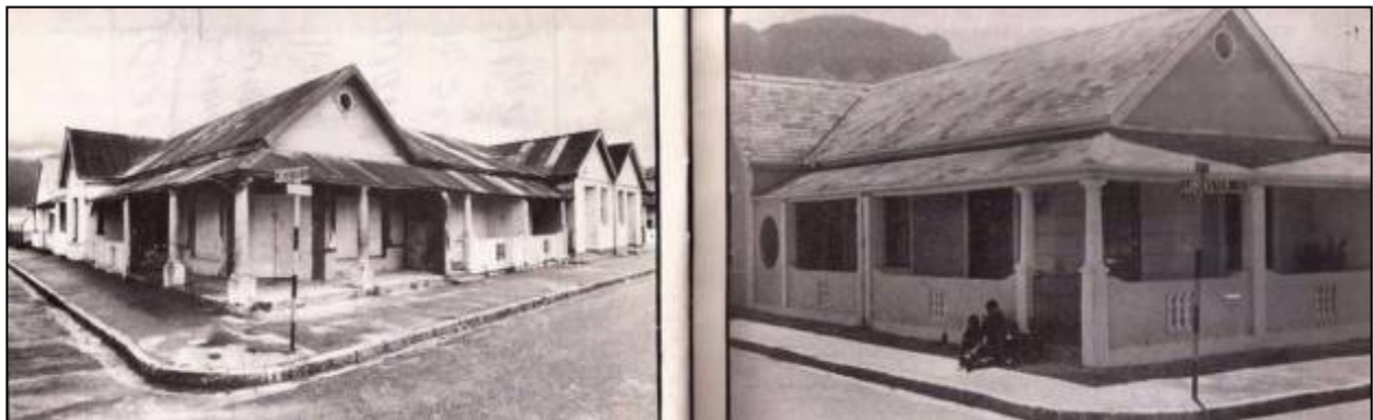
Figure 4.15: House on the corner of Lancaster St and 2 nd Avenue before evictions (left) and after gentrification. It is currently a dentist's office (Source: UWO, 1982).
