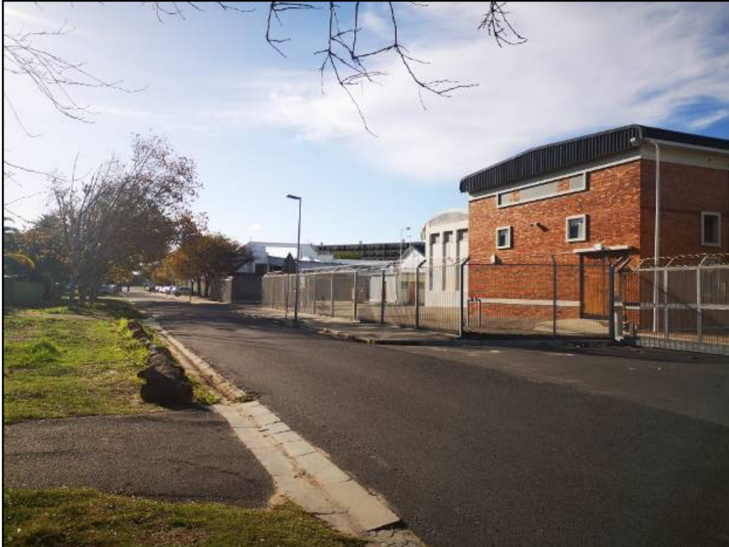
Photograph 4.55: City of Cape Town substation located to the south of Master Cars facilities.
