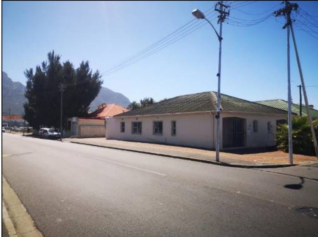
Photograph 4.9: Property located at intersection with Franklin Road
