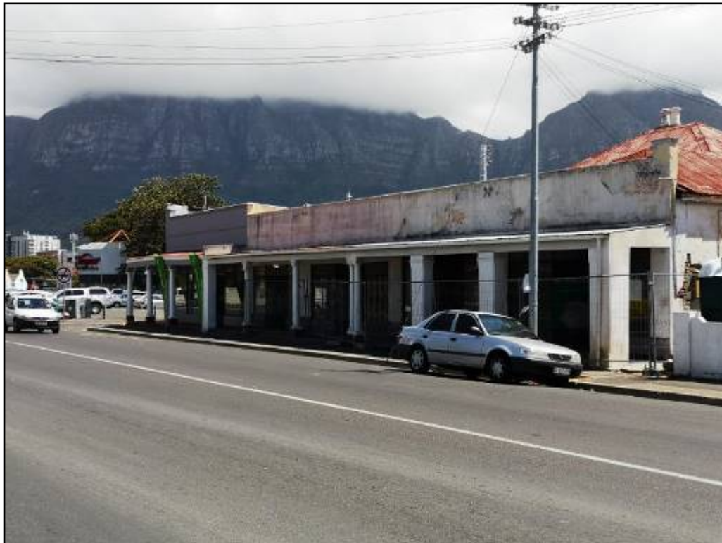
Photograph 4.28: Vacant properties owned by the CoCT
