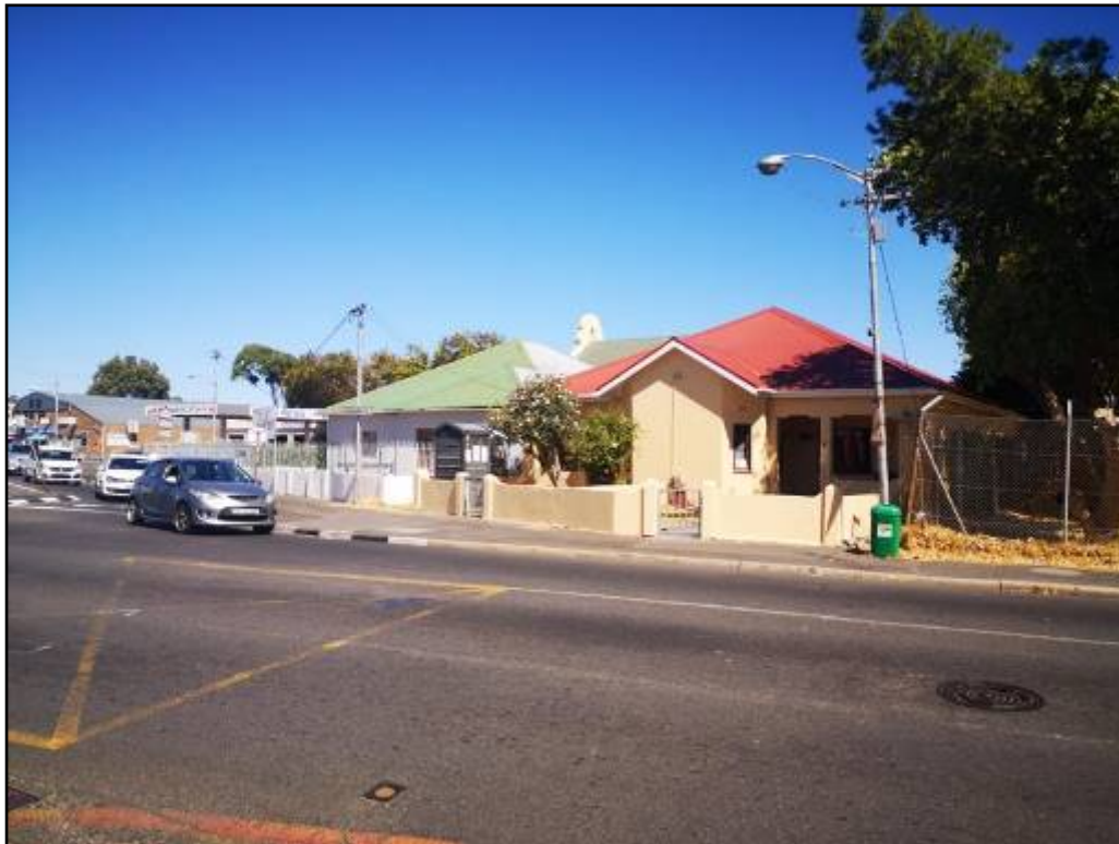
Photograph 4.22: Erf 53509 (red roof)
