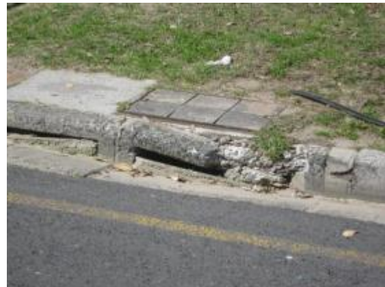
Figure 18 Road kerb inlet grid requiring replacement
