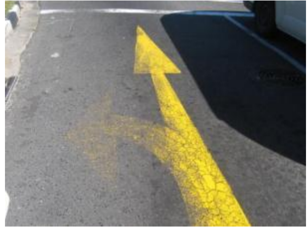
Figure 20 – Street marking signs needs repainting
