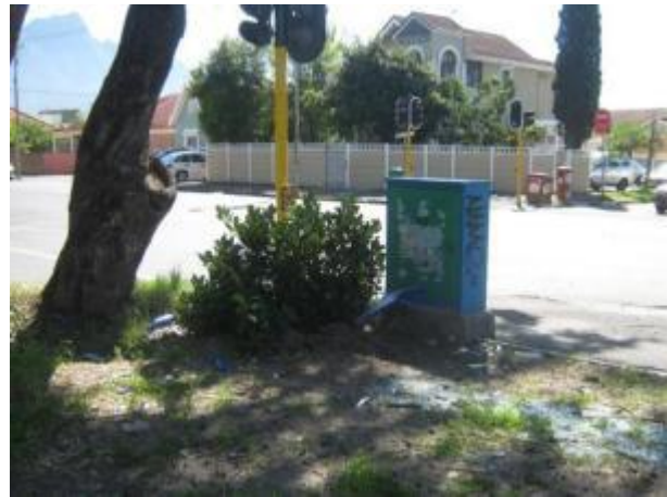
Figure 22 Illegal posters on Telkom signal box with graffiti
