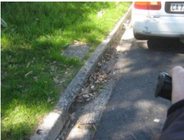
Figure 27 Partially blocked kerb inlets
