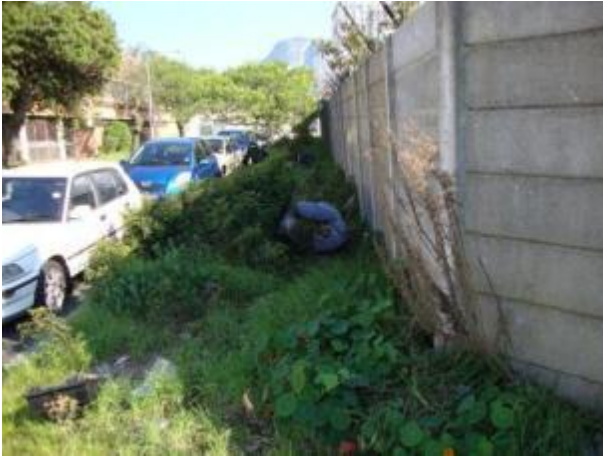
Figure 19 Sidewalk requiring rehabilitation, garbage prevalent.
