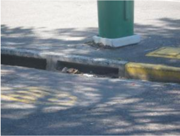
Figure 29 - Partially blocked kerb inlets
