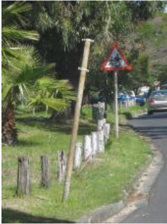
Figure 23 Neglected road signs and fencing
