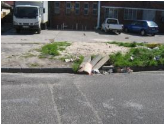
Figure 17 Road kerb inlet grid requiring replacement, leaking sewerage evident.
