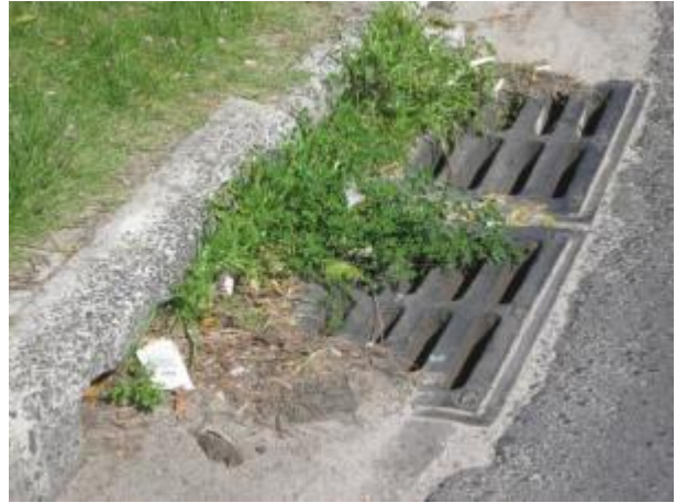
Figure 30 - Partially blocked kerb inlets
