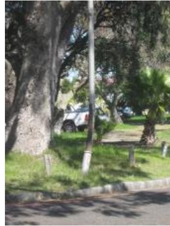
Figure 24 Lighting poles poor condition
