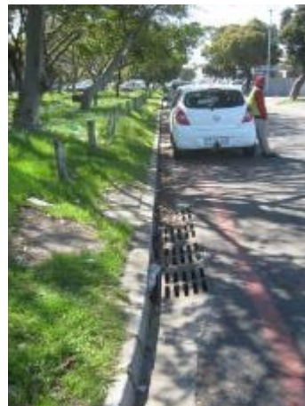
Figure 28 - Partially blocked kerb inlets
