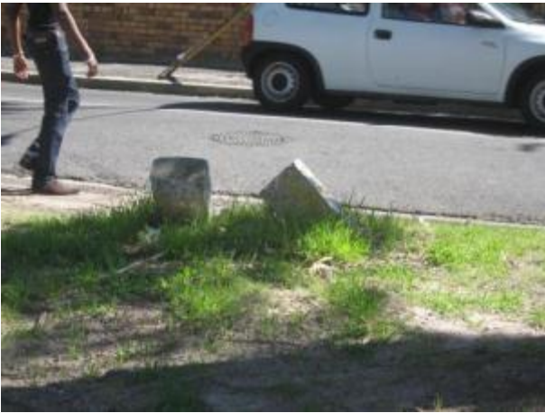
Figure 25 Bollards broken
